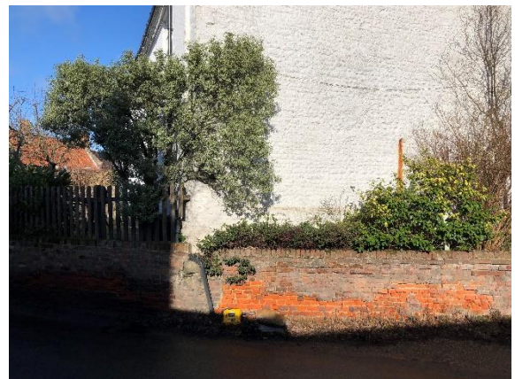
Figure 3.9: Vibration Monitor at Whitehouse Farm
